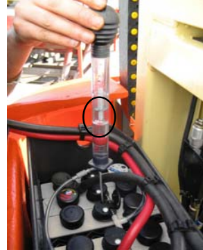
Figure 8-4. Measuring Electrolyte Specific Gravity
